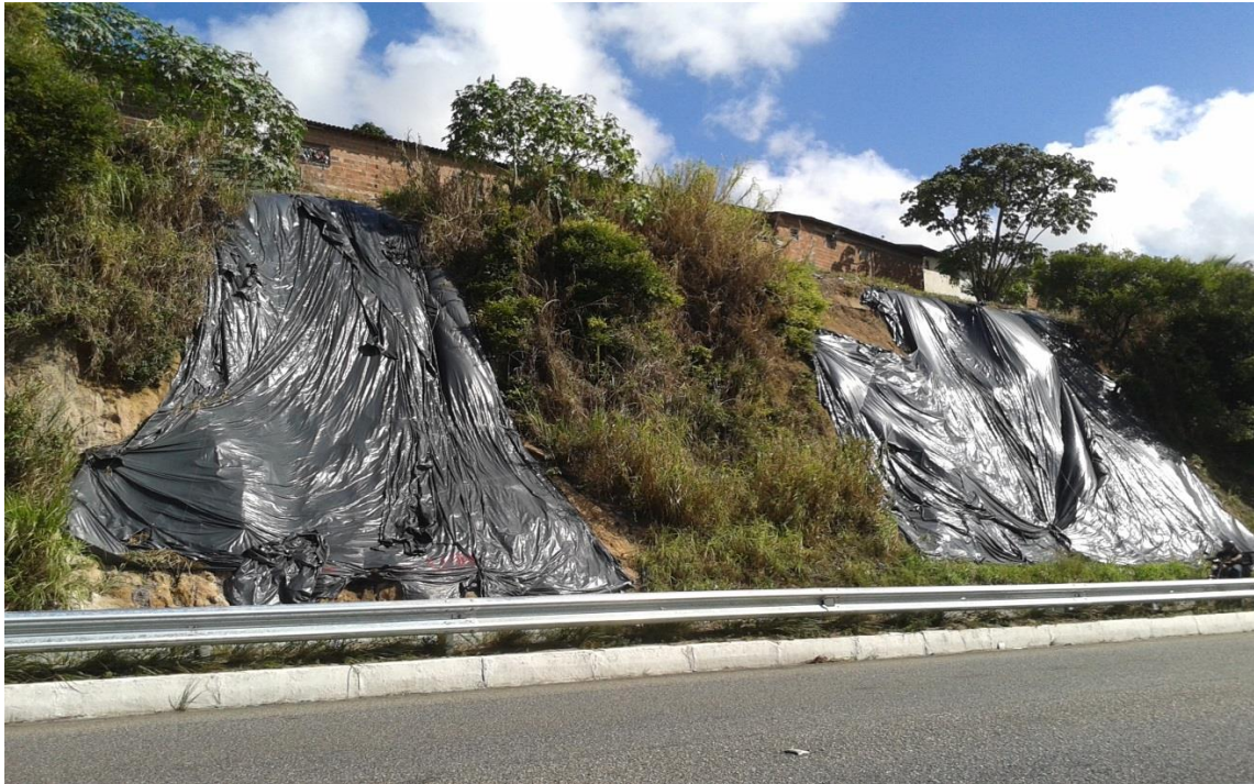
Figura 20 – Lona protegendo as encostas
